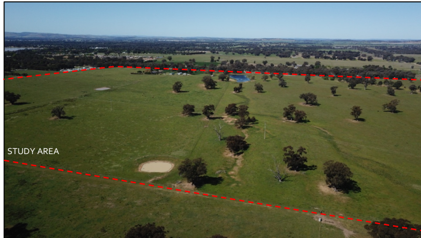
Photo Point A5. Looking east at 456 – 475 Plumptton Road, Rowan, the Study Area showing the extent of internal and surrounding hazard vegetation.
