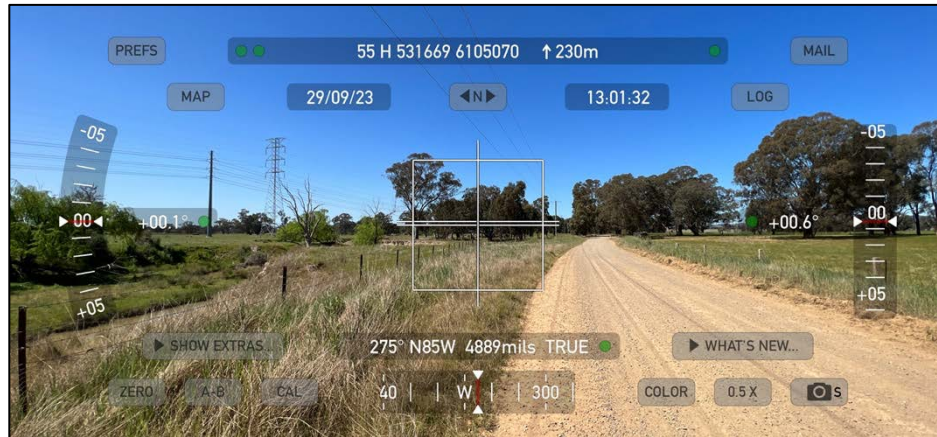
Photo Point 13. Showing the general condition of the well-maintained Rowan Road and hazard vegetation south of the Study Area.
